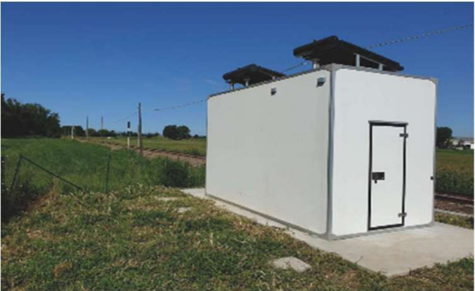
LEVEL CROSSING (PL17) in Cavriago (RE - IT) FER Railways
