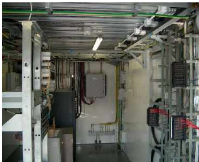
Floor mounted Racks (direct screwed on the floor)
