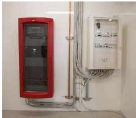
Wall mounted panels (direct screwed on the wall)
