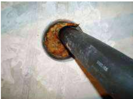
Foamed pipe / sleeve (ARAMCO)
